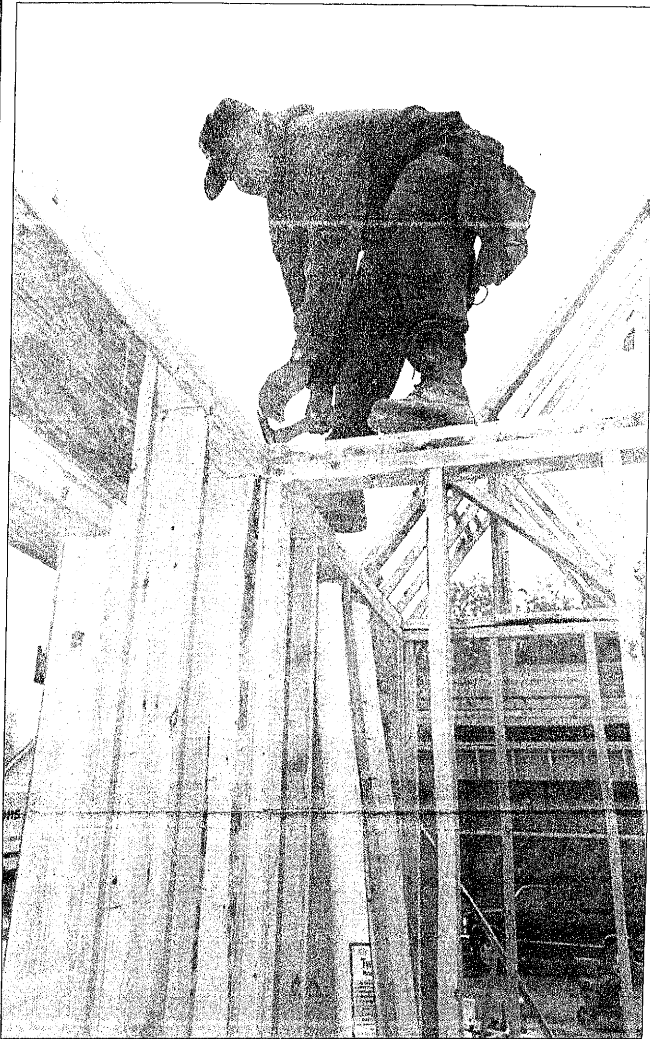
Above: Rougher Clinton Williams, balancing on the partition wall of a home under construction, works on nailing together support beams.
