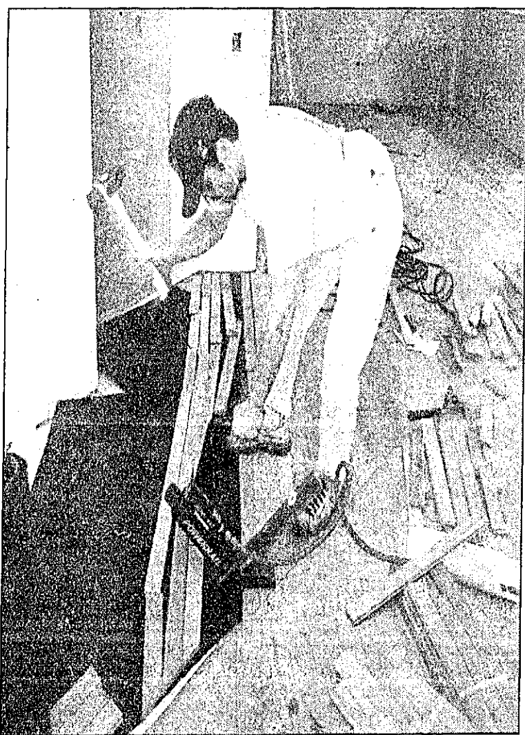
Above: In Abbey Hills, the wood floor is laid in place by an employee of the flooring subcontractor. Left: Finish carpenter Greg Sturgeon works on putting in the closet's folding doors.
