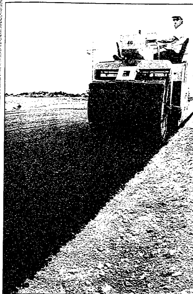
A worker from DPC Asphalt smooths paving for Taft Road.
