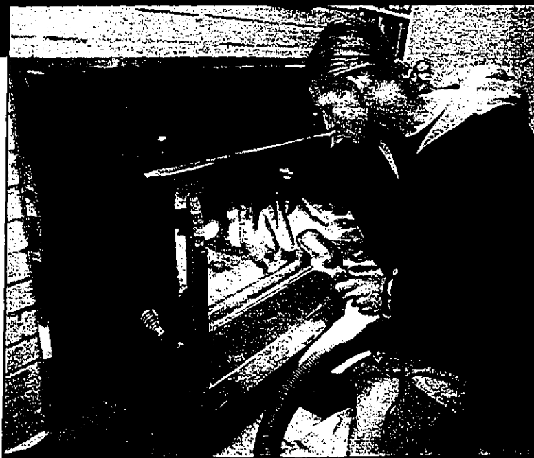
Above: In traditional garb, Don Morgan of Alpha and Omega Chimney Sweeps pulls a flue-brush out of a Northville chimney along with a puff of creosote.
