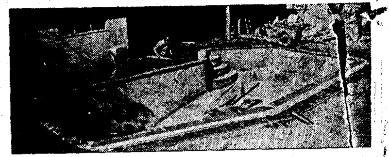
Workers pour concrete apron as a finishing touch after swimming pool itself has been completed. The pool also is concrete, sprayed on by Gunitite process.
