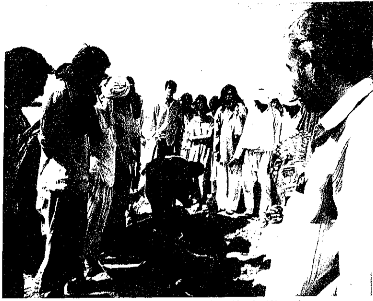
Everybody takes turns digging for Sursardham ground-breaking for 121 new houses.
