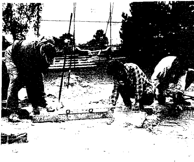
NABF volunteers Carl Galletti (left), Cathy Galletti and Ron Angove work at getting clay put down as a base under the batters' boxes at Hillside field.
