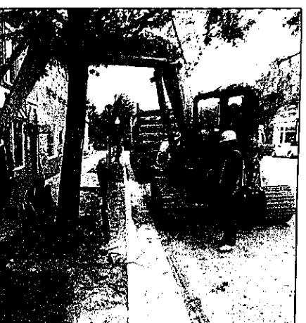
Downtown Milford will see the cranes move from the tending to the sidewalks, as seen here during the brick paver project, the Main Street itself this month.
