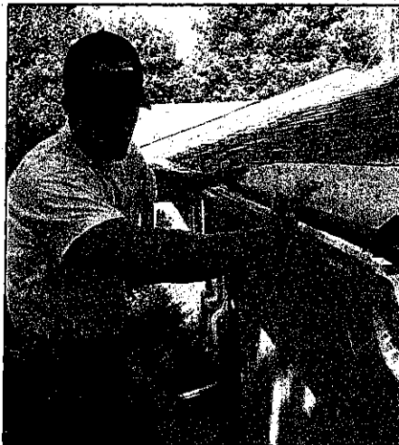
Above, Atlas Gutter Helmet Installer Doug Bennett prepares sections of the Gutter Helmet for installation. Then, at left, Dave Calvin fits the Gutter Helmet to the roof of a home.
