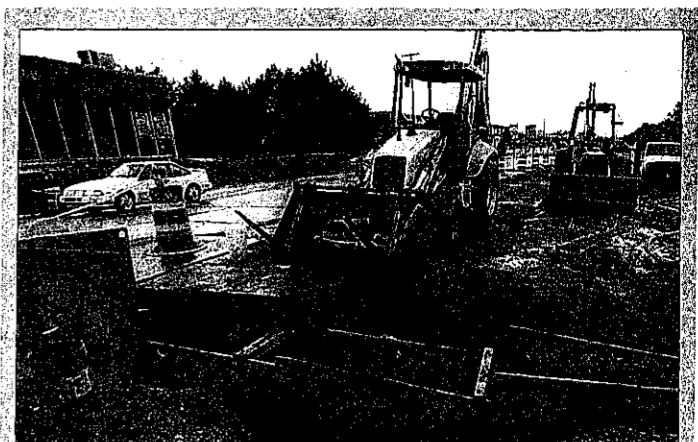
Work continues last Friday afternoon by Detroit-Edeon personnel to place a utility line underneath Twelve Mile Road at Novi Road. The busy intersection was closed to allow safe completion of road improvements.
