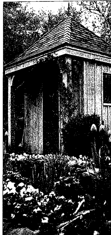
Fred Murray had his 9-foot by 9-foot cedarboard and batten garden shed built at his home about five years ago. The door seen here is actually an antique that used to be on another house — it still has the old address on it — but now is just decorative.
