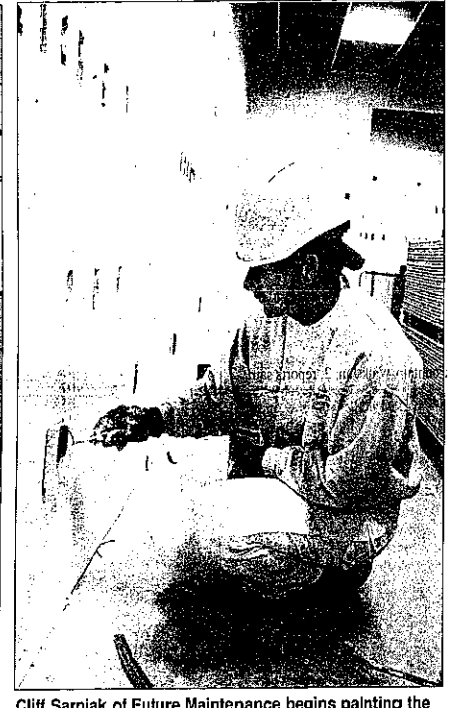
Cliff Sarniak of Future Maintenance begins painting the walls of the Providence Park Hospital surgery patient prep area. The hospital will open this summer.
