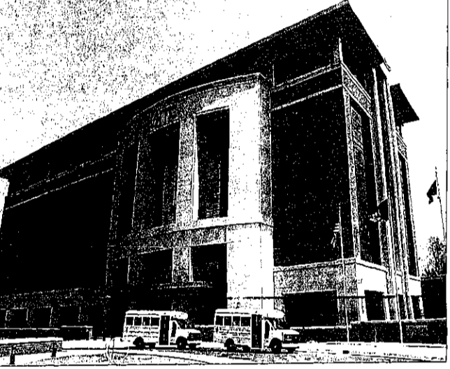
ITC's new Novi campus and its six-story building, which can be easily seen from the Michigan 5.
