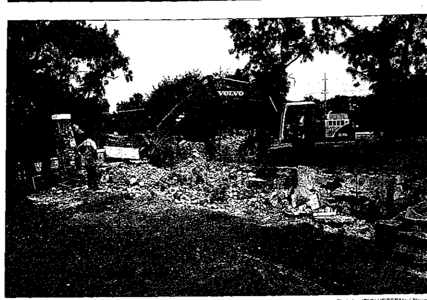
The former Fuerst Farm home is torn down on Tuesday, Aug. 19. By 10 a.m., the only discernible part of the home that remained was a single stone support column, at left, that used to hold up the front porch roof.
