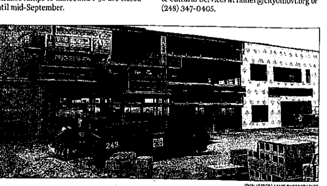
Brick by brick The exterior of the new Novi Public Library is being cinderblock in this photo from July 2009.
