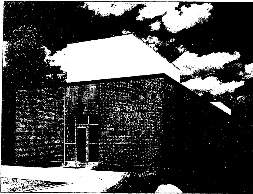
The Firearms Training Center in Novi opened in 2008 and was funded using federal drug forfeiture funds as a result of Operation Falling Star. The police department is currently in negotiations with representatives from the Customs and Border Patrol to possibly rent out the facility on a regular basis.
