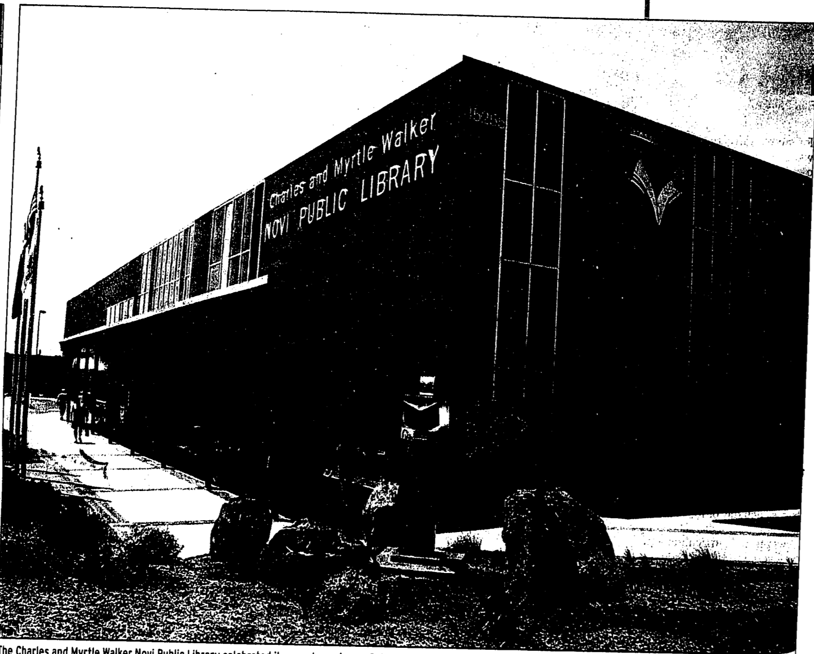
The Charles and Myrtle Walker Novi Public Library celebrated its grand opening on Saturday. The library opened to the public June 1, and was completed on time and under the $12.5 million budget voters approved in 2007.
