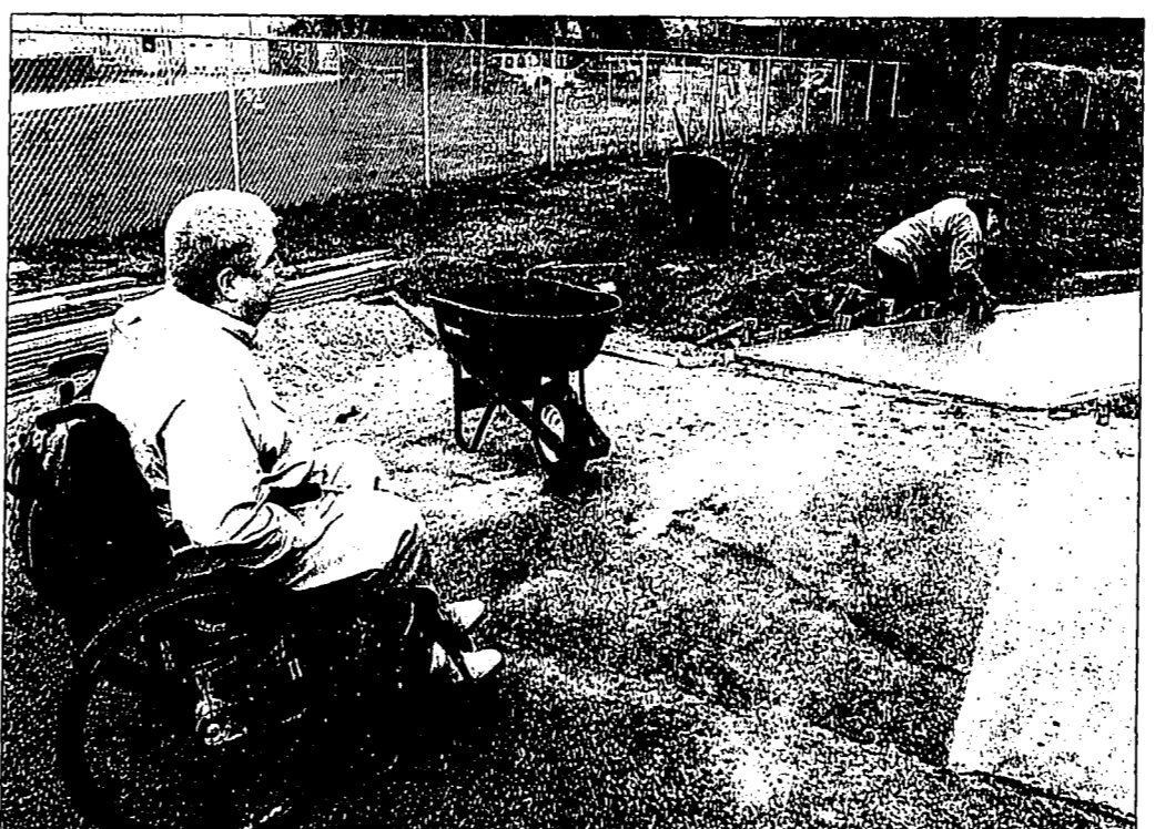
Michigan Paralyzed Veteran's of America executive director Mike Harris surveys the widening of a sidewalk leading into the non-profit organization's Grand River Avenue building.
