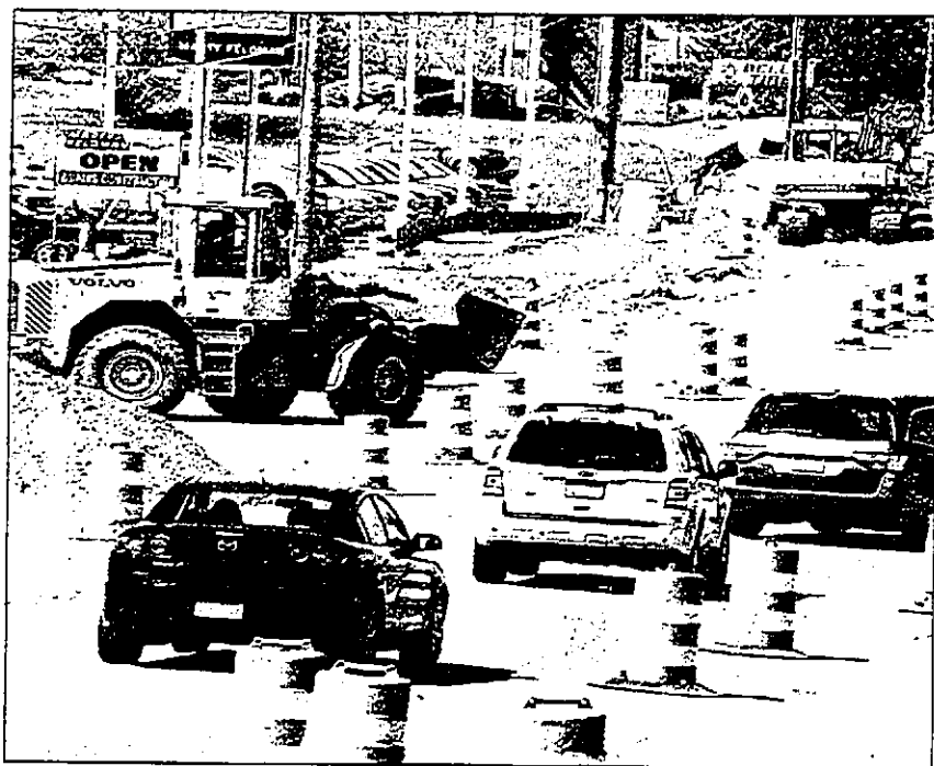
Repaving work begins on Grand River Avenue west of Meadowbrook on April 6. The project, costing about $4.1 million, should be finished by mid-September.
