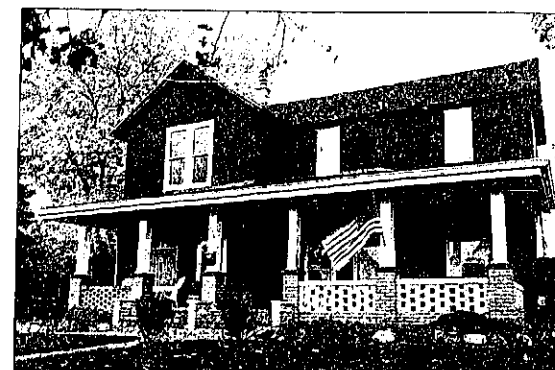
This house on Starkweather in Plymouth had long been a two-family dwelling until Scott and Alison Jones planned to make it a single family home again. A recent Fannie Mae survey revealed some encouraging signs in the housing market.
