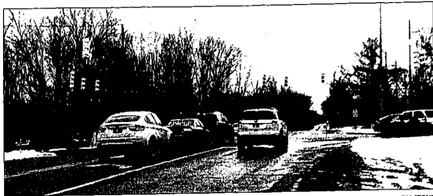
Improvements to Eight Mile Road (shown fading west) include repaving and bike lanes on each side to Napier Road as well as pedestrian improvements at this intersection at Beck Road.
