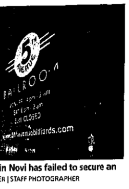
The owner of Fifth Avenue in Novi has failed to secure an occupancy permit. JOHN HEIDER/STAFF PHOTOGRAPHER
