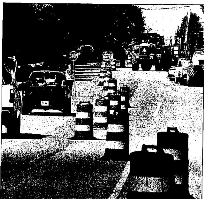
One of the delays affecting Northville and Novi commuters is a road-widening project being carried out along Eight Mile Road west of Beck. Drivers will find slow going as the road is pinched down to a single lane. JOHN HEDDER | STAFF PHOTOGRAPHER
