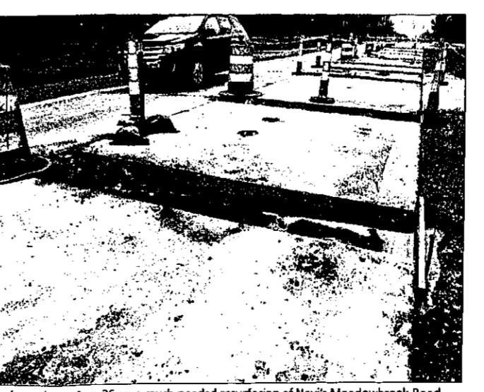
Work continues Aug. 26 on a much-needed resurfacing of Novi's Meadowbrook Road between Nine and 10 Mile. The road is currently only running in one direction, north, although access to all the businesses along Meadowbrook is being maintained. JOHN HEDER | STAFF PHOTOGRAPHER
