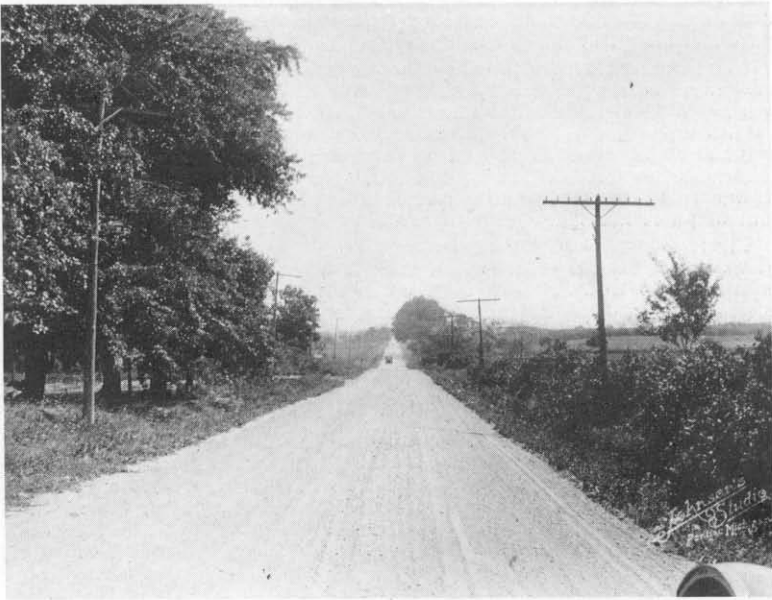
A gravel surface well maintained provides a good road for light traffic. West Rochester Road, Avon Township.
