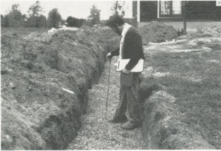
The sewage disposal field is inspected.
