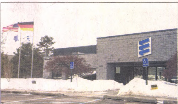
Eberspaecher's North American facility, at 43700 Gen Mar, off Novi Road, petitioned the city to allow it to load and unload tractor trailers outside of the time normally allotted for that activity. JOHN HEIDER | STAFF PHOTOGRAPHER
