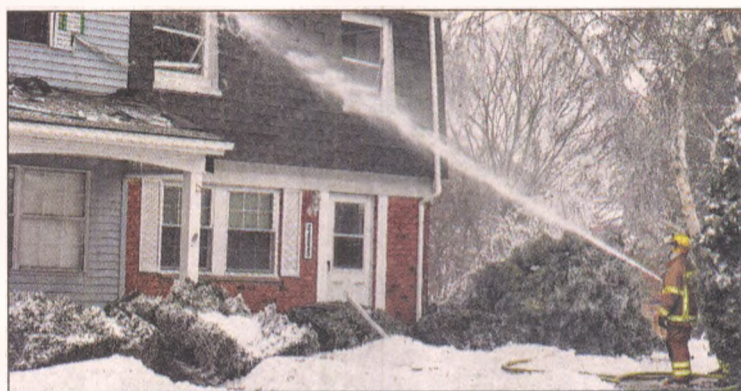
Novi firefighters work on tamping down a hot spot as they continue efforts to extinguish a fire that destroyed six units of Olde Orchard condos March 12. The fire, which began in the morning, destroyed all six units and slightly injured one female occupant with minor burns. JOHN HEIDER | STAFF PHOTOGRAPHER
