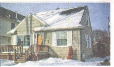
OPEN 1-4 | 1303 Cole Street, Birmingham - Location! Walk to Downtown and the Rail District from this charming bungalow. $192,000 Joanna Drukker (248) 639-4903
