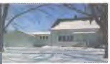
OPEN 1-4 | 46759 Vineyard, Shelby Township - Look No Further! This gorgeous home is loaded with updates. Refinished hardwoods. $149,900 Becky Livernois (248) 817-4554
