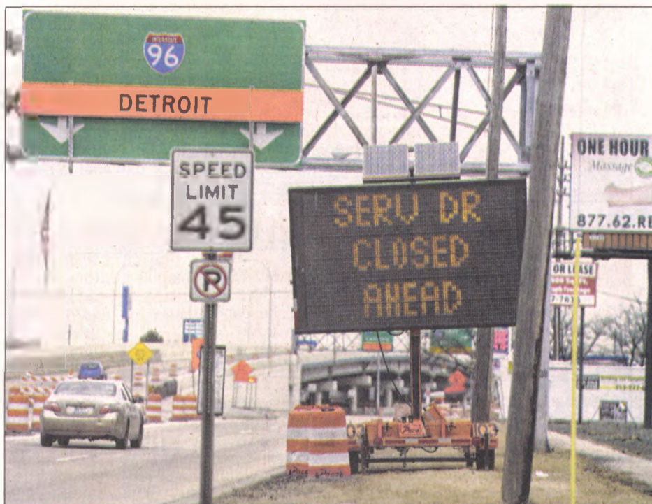
Traffic is diverted to the Schoolcraft service drive Monday for work on I-96 that has the freeway closed from Telegraph to Newburgh until October. MANDI WRIGHT | GANNETT MICHIGAN
