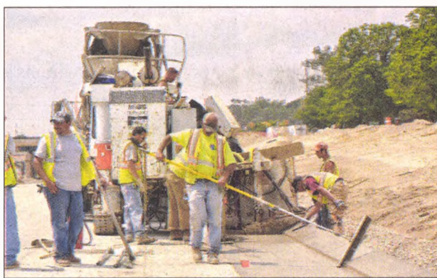
The concrete shoulder is formed and finished. BILL BRESLER | STAFF PHOTOGRAPHER
