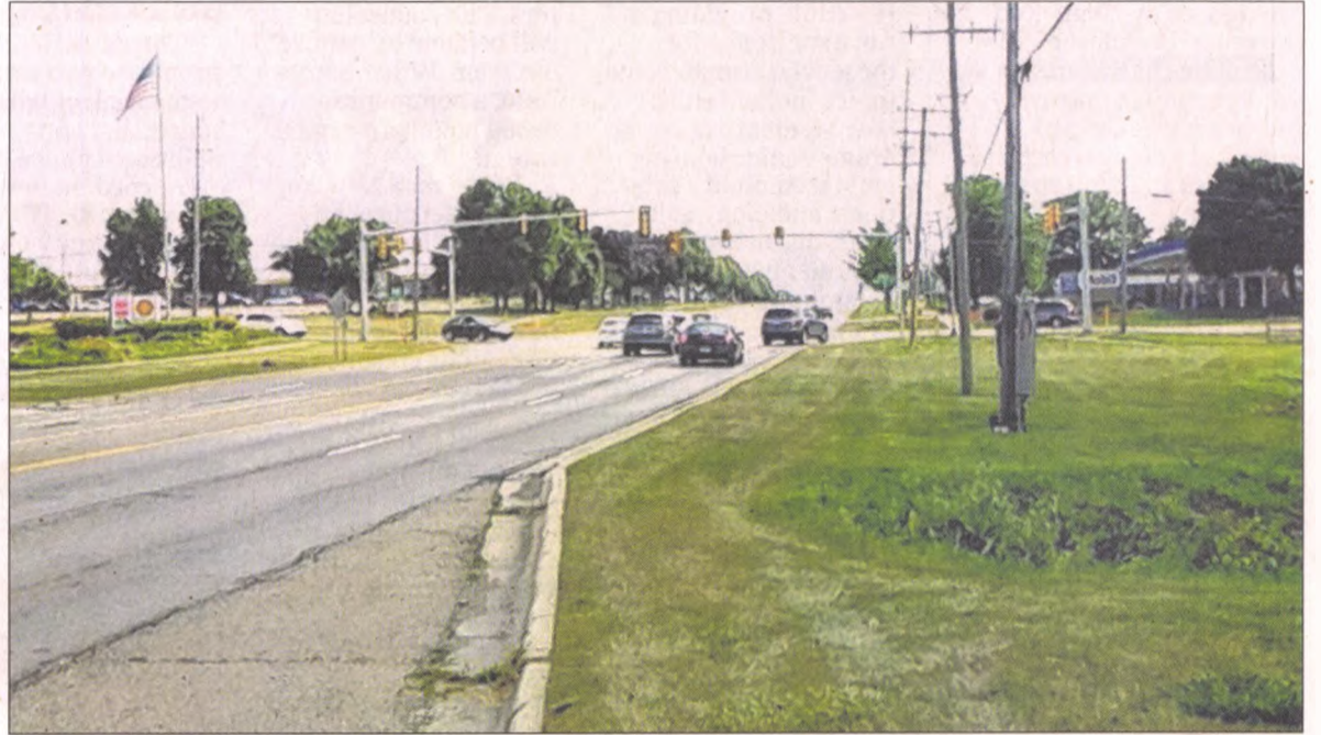
For southbound Haggerty Road drivers turning right on to Grand River Avenue, a right-turn lane will be installed where grass is currently. The angled curb pictured is the exit of the Mercedes-Benz of Novi dealership.
