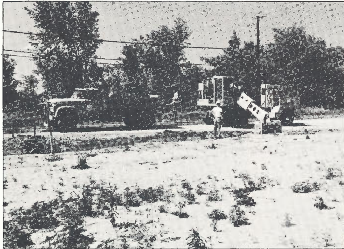
Ditch Cleanout Operation
