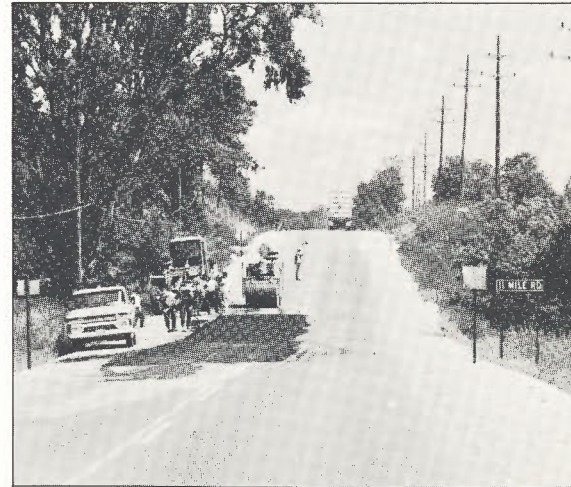
Bituminous Concrete Patching
