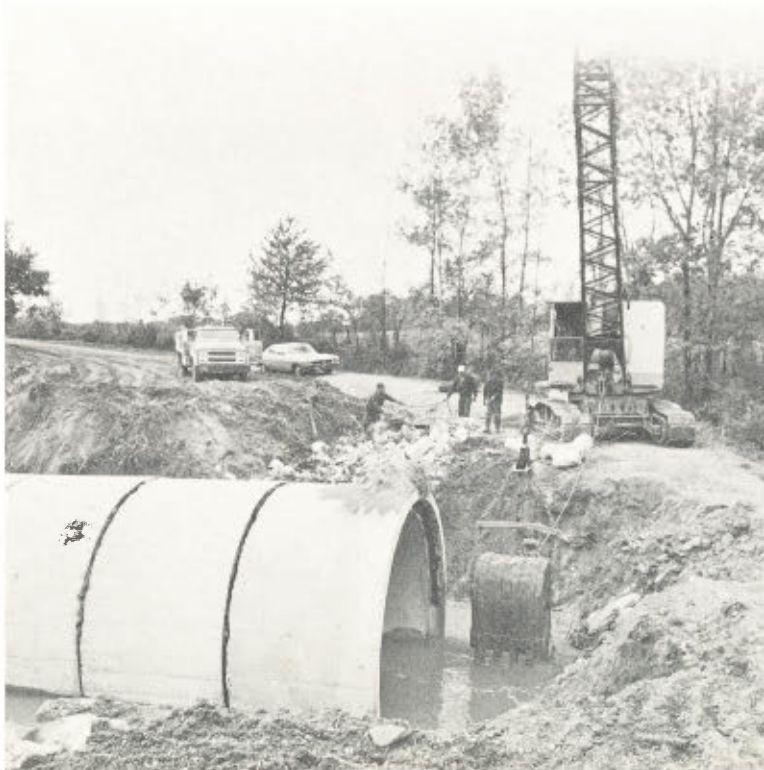
Maintenance forces replacing rural area bridge.
