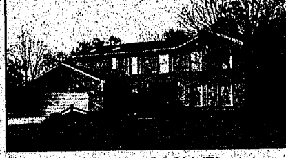
PREMIUM SITE & POOL! Elegant and prestigious! Gourmet kitchen opens to family room with fireplace, 12x17 sunroom overlooking wrap around pool with spa. Formal dining room with hardwood floor, lavish master suite with 3 closets, bath with jet tub! $319,977 (47TIM) (248) 652-8000
