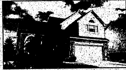
MOVE IN and enjoy this spacious 4 bedroom, 2 1/2 bath Colonial on premium landscaped lot with C/A, sprinklers, gas fp, hdwd floors; crown moldings, neutral T/O. Many upgrades: carpet, lights, daylight basement, 1st fl laundry, deck. Sub offers community pool, bike trails. $249,900 (48BRI) (248) 652-8000
