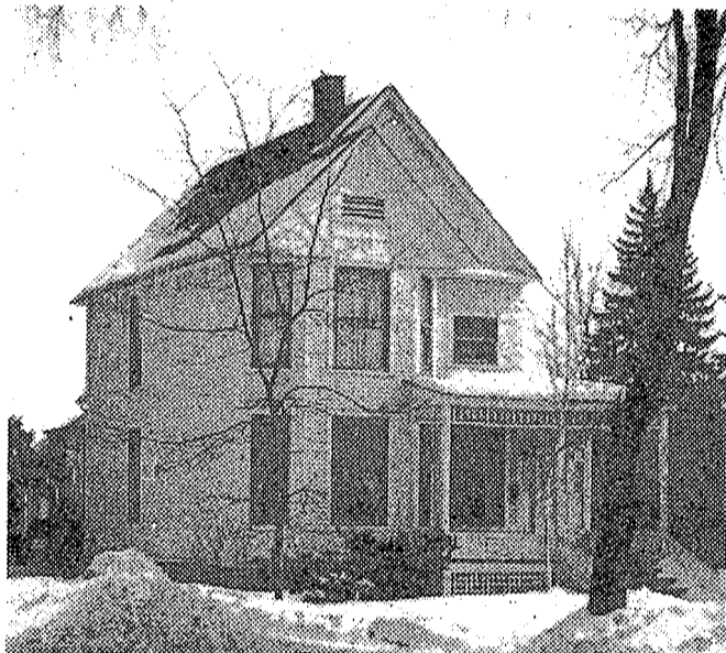
This Clarkston home, built in 1884, has horizontal bands of spindlework on the front porch. The steep roof, wide eaves, and two-story bay are also typical of Queen Anne as well as Stick style. The overlaid sticks in the gables, while seeming to relate to the structural elements [as in Stick style], may have been meant to simulate half-timbering, an English detail often used with Queen Anne.
