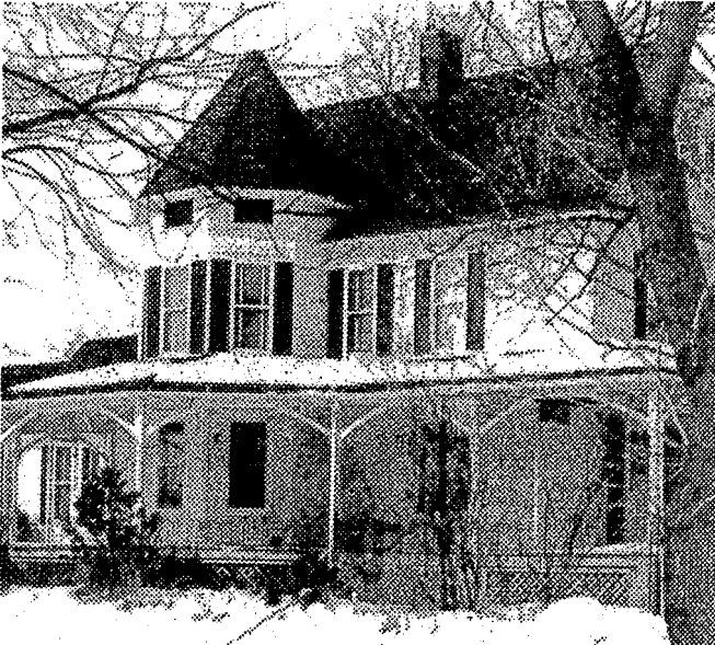
Built in 1908, this large home on Main Street has changed very little since that time. Another example of Queen Anne, it has an irregular plan with a high steep roof, a turret, wide verandas, and a bay window on the third story in the front. Scalloped shingles and latticework provide a contrast to the horizontal clapboard.
