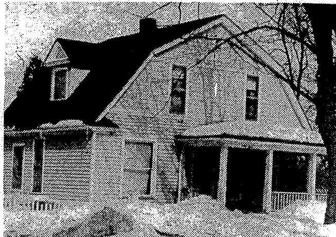
This home on East Washington, built in the 1890s, shows the influence of the Queen Anne style. The wide veranda extends along two sides of the house. The scalloped shingles contrast with the horizontal clapboard on the first floor. The gambrel roof, with dormers, allows for increased space on the second floor.
