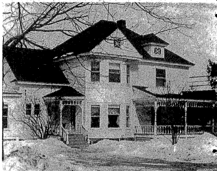
This side view from still another Queen Anne house, this one on the corner of Main Street and Miller Road shows the delicate spindlework which is typical of the style. Other important characteristics include the irregular plan, multiple roofs with dormers, a variety of textures [shingle and clapboard], a two-story bay window [another in the front of the house], and a variety of window shapes. All provide a picturesque effect.
