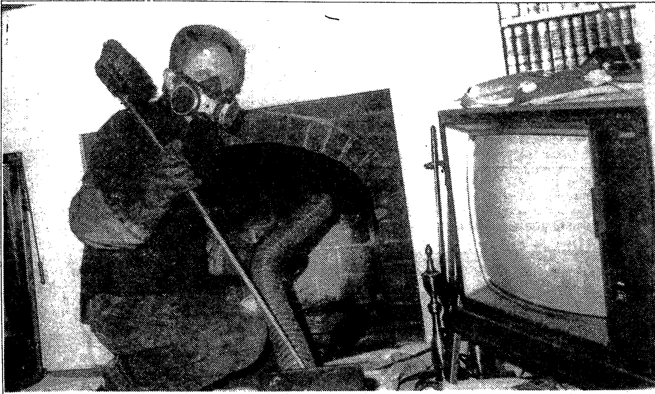
After sweeping from the top of the chimney, Master Sweep, Jim Rutledge once again cleans the firebox. The mask, trouble light, and vacuum enable Rutledge to do a thorough job.
