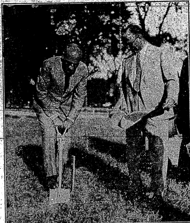
It looks as though Gov. Comstock, posing with James B. Jones, president of the State Fair Association, was digging for worms, but he's not. The governor is merely turning the sod for the free model house that will be built on the State Fair Grounds, Detroit, for the 1934 Fair, August 31 to September 9. The home will be fully decorated.
