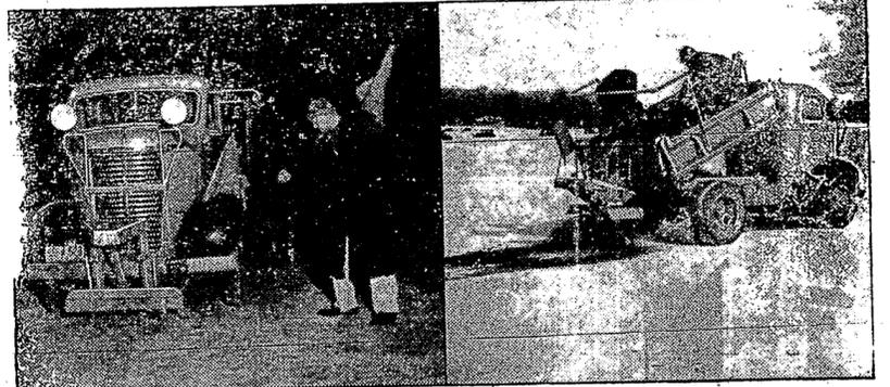
Left: 3,000 individual tests were made during the investigation of winter driving hazards, some of them being conducted at night. Right: Treated abrasives were spread on the frozen lake surface and demonstrations made of their effectiveness in skidproofing.
