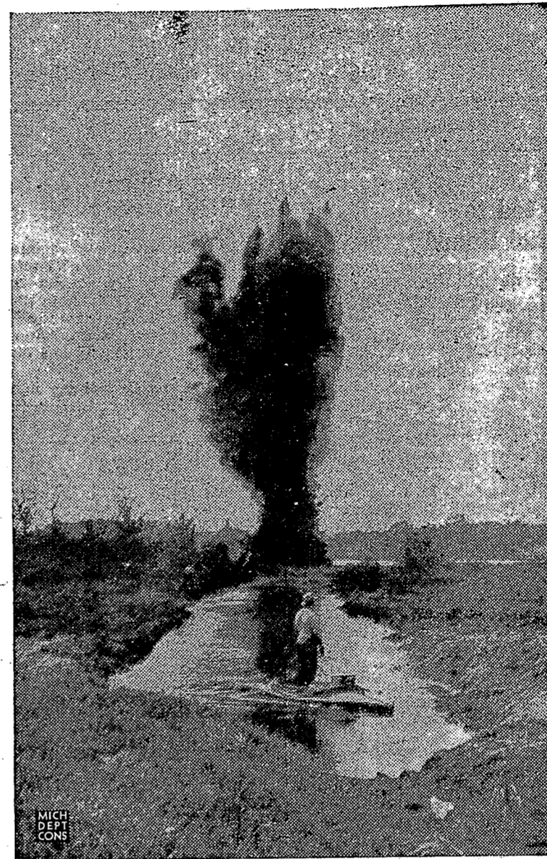
Tossed 200 feet into the air by a charge of dynamite are tons of swampland and floating bog that barred the last stretch of a boat channel dug with explosives from open water through 600 feet of marsh to solid ground at the public fishing site on the shore of Big Crooked lake, in Livingston county.
