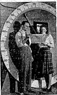
How does heat affect your automobile engine? This huge test engine thermometer developed by Gulf research at Mellon Institute is helping find the answers. The apparatus gives quick temperature data for as many as several hundred points on a battery of laboratory test engines used in fundamental studies of fuel and oil behavior. An engineer here shows a laboratory assistant the mutiple temperature record taken in tests run on a single engine.
