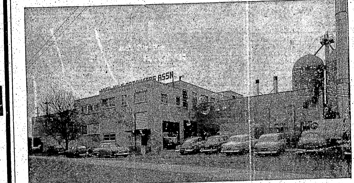
Exterior of the new main plant of the Michigan Milk Producers Association at Imlay City.
