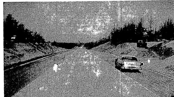
Five miles of new 22 ft. concrete pavement 8 inches thick, reinforced with steel, from Grayling south on US-27 was opened to traffic on Decem-
