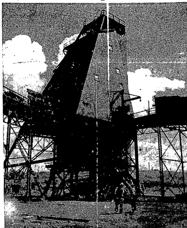
This shafthouse over one of Michigan's western upper peninsula iron mines is a standing symbol of an industry that for years has been the backbone of the state's mining industry. Each year, nearly 100,000,000 tons of ore come down the Great Lakes from the western Lake Superior region.
