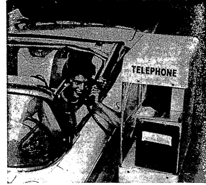
Mrs. Norma Gilbert stops to use the newest type of outdoor phone booth which the Michigan Bell Telephone Company has installed on an experimental basis on US 10, north of Pontiac. This boothette allows the motorist to phone from a car while still sitting in the driver's seat.
