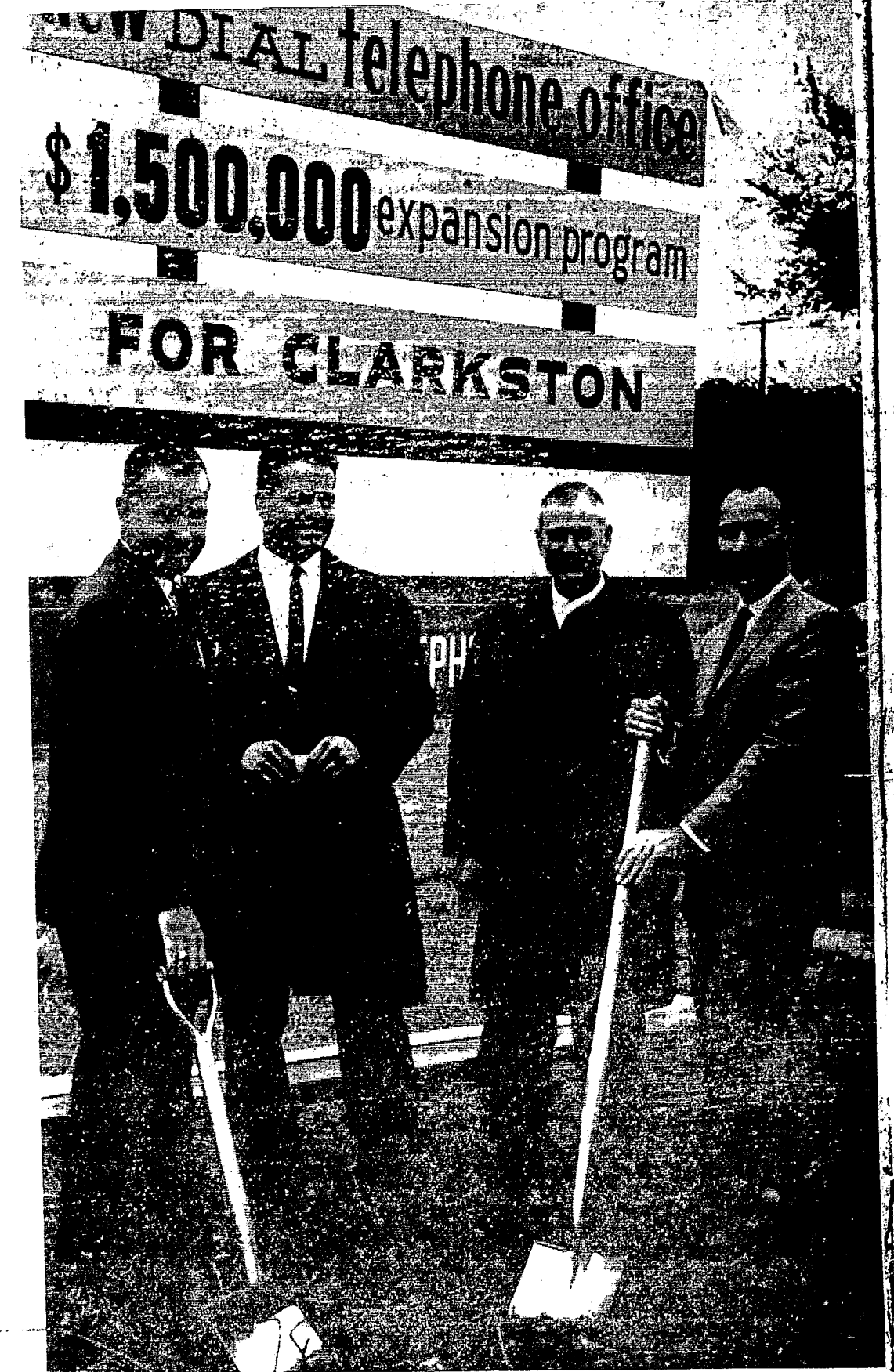
Clarkston Village President, James Huttenlocher (left) and Independence Township Clerk, Howard Altman, right are shown breaking ground for Clarkston's proposed telephone office as two telephone representatives Eugene Russell, (left) and Charles Woodhead supervise.
