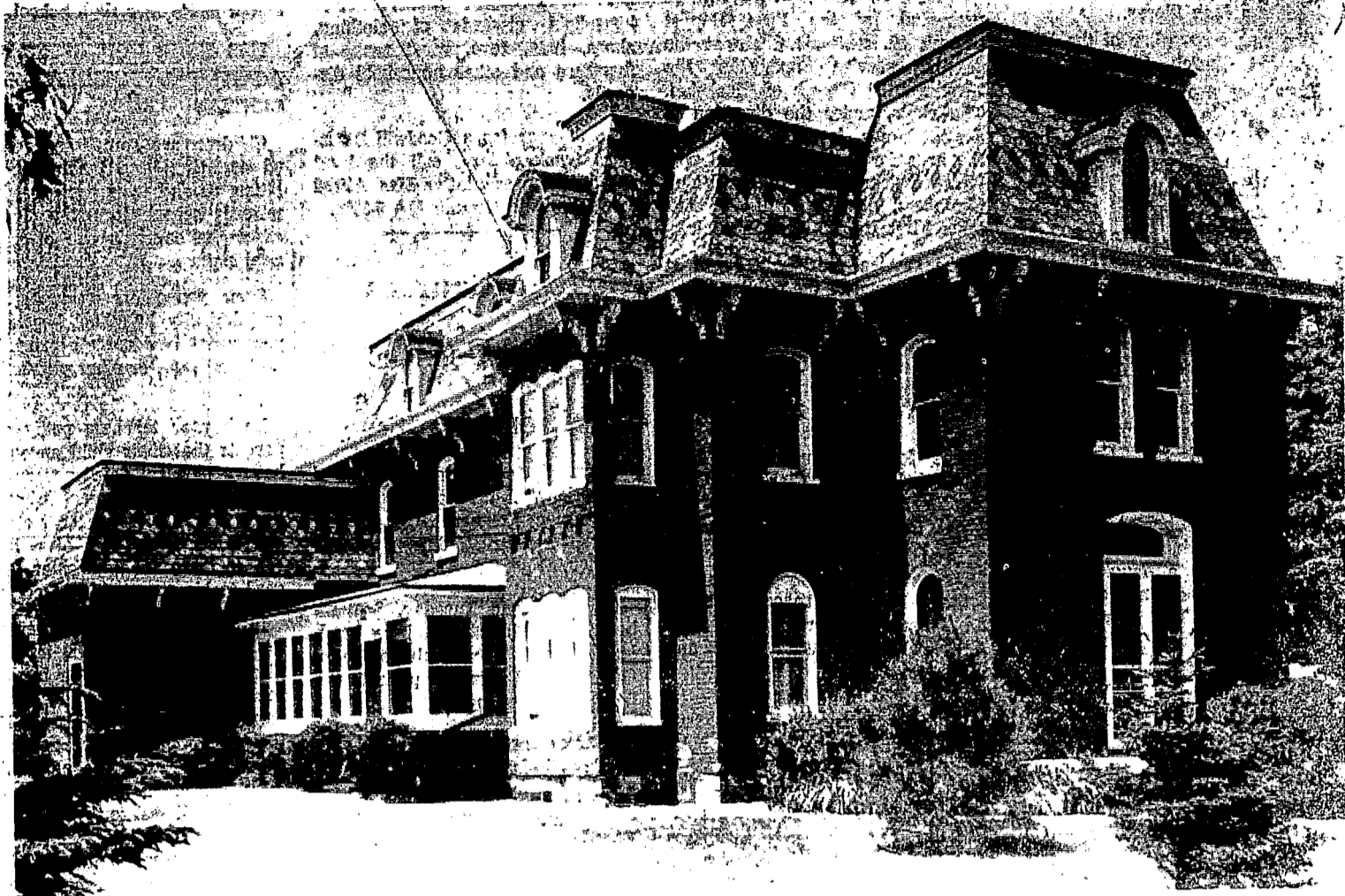
The pride of the Samuel Miller, Jr. family is this staunch eighteen room home built by Mr. Miller's grandfather and maintained in perfect
