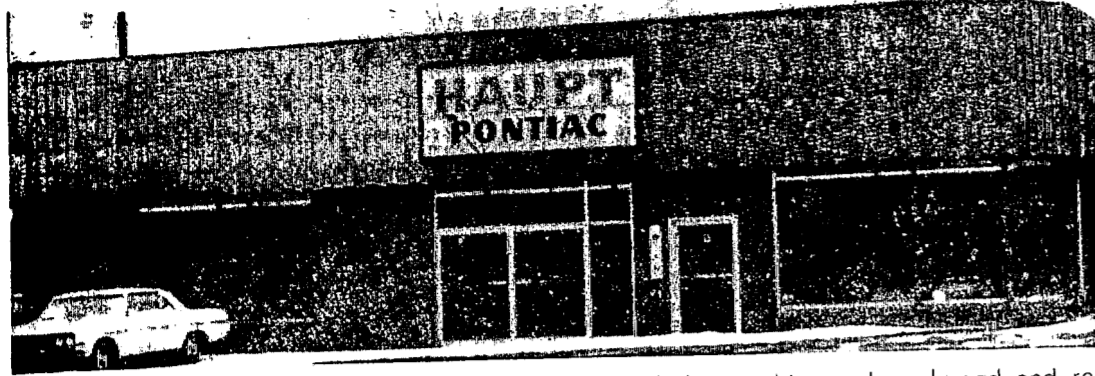
ANODIZED ALUMINUM in an attractive gold color accents the new front section of Haupt Pontiac's new addition. Located north
