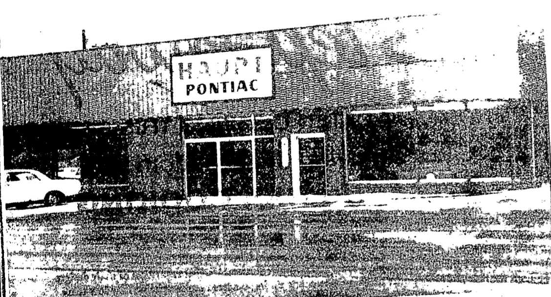
Anodized aluminum in a gold color accents the front of our remodeled Showroom
