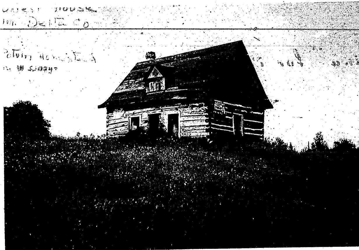
Cabin of earlier days but much larger than most—loft window was long to make it easier to store bundles of hay, etc. from the outside. (Gift of Marquette County Historical Society) Courtesy Michigan Historical Commission
