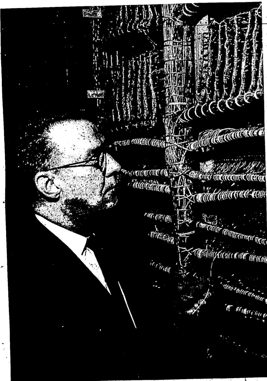
MAZE OF WIRES-For every telephone there has to be a pair of wires running from the station to the phone. One of the wires is held by Duane Hursfall. There are 3,000 of them in the large cable in the center. The Clarkston facility handles only the 625-exchange.
