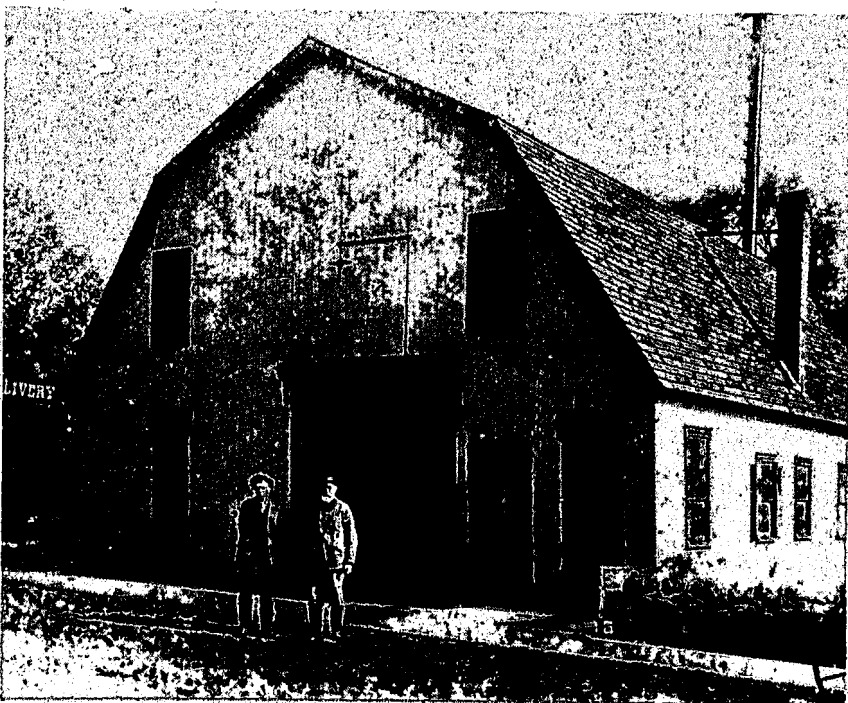
Linabury's Livery stood on the east side of Main Street near the Clinton River. Part of that stone fence still stands today.
